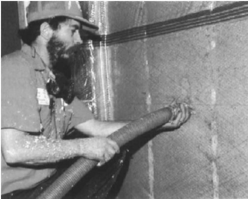
Figure 7.11 Installation through vapor retarder. ( ParPac, Inc. )
