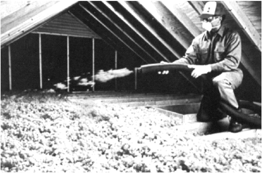
Figure 7.1 Blowing loose fill insulation. (NREL/DOE)
