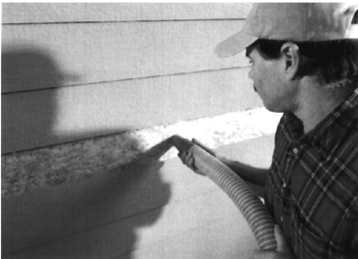
Figure 7.3 Cellulose installation by pneumatic equipment. ( Greenstone )
